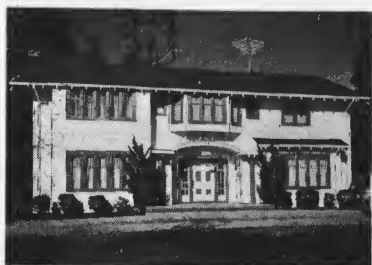
LOOKS LIKE WOOD, but the clapboard look on the exterior of this home is actually vinyl siding with "wood-grained" finish. Vinyl siding is maintenance free, and is guaranteed for 20 years.
